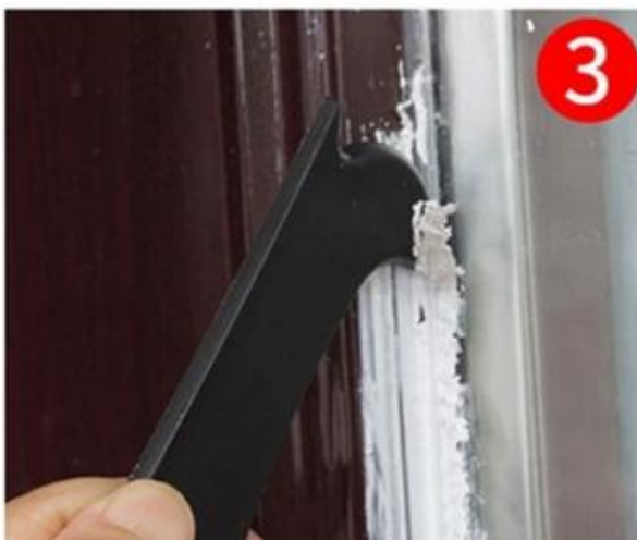
Gently pull with a sharp corner to scrape off
