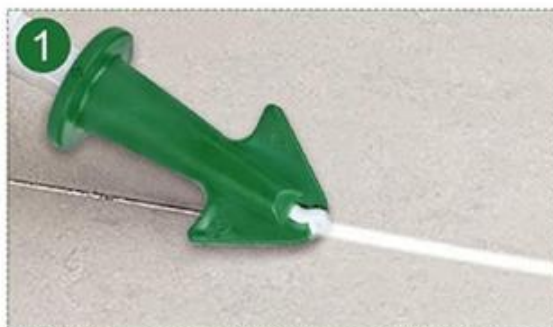
1 Pushing silicone caulking gun smoothly
