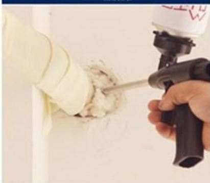
Repair air conditioning holes.
